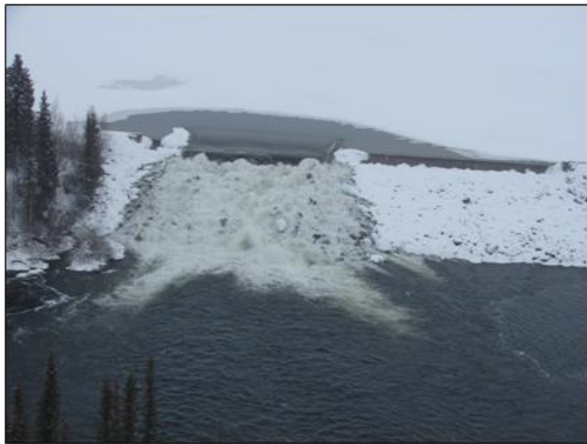
Emergency spillway under high flow conditions in the fall of 2008
