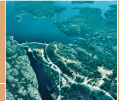
Aerial photo of the Ted Humphry's Plant at Snare Rapids.
