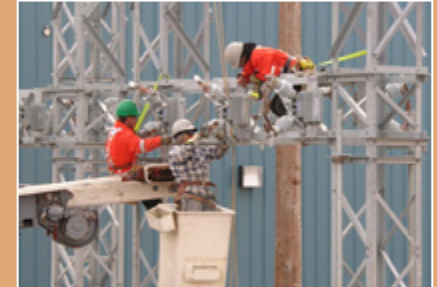
25kv Upgrade of Inuvik Substation - Summer 2005
