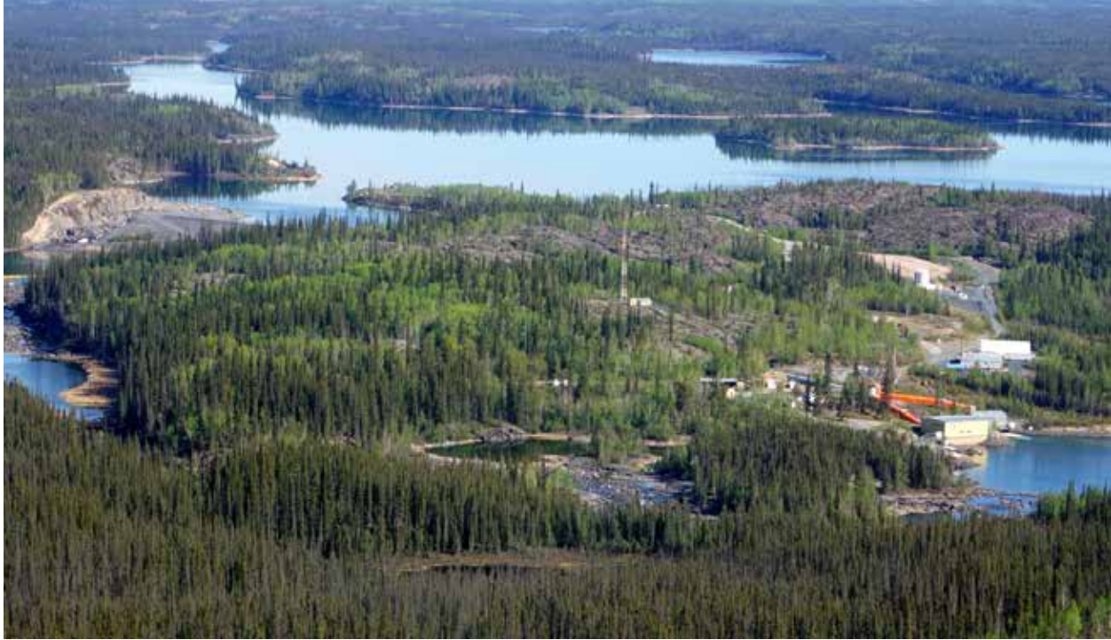
Bluefish Hydro Generating Facility
