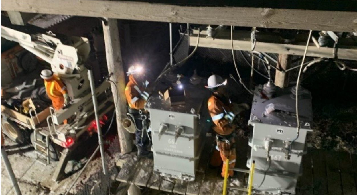
Our team responds to all problems, regardless of the time or weather conditions. In this photo, linepeople are replacing three feeder transformers in Tuyktoyaktuk. The salt air in coastal communities causes corrosion (rust) to occur more quickly than in other locations.
