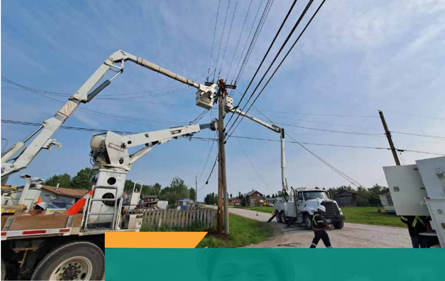
Maintenance of distribution lines and power poles is an ongoing activity.
